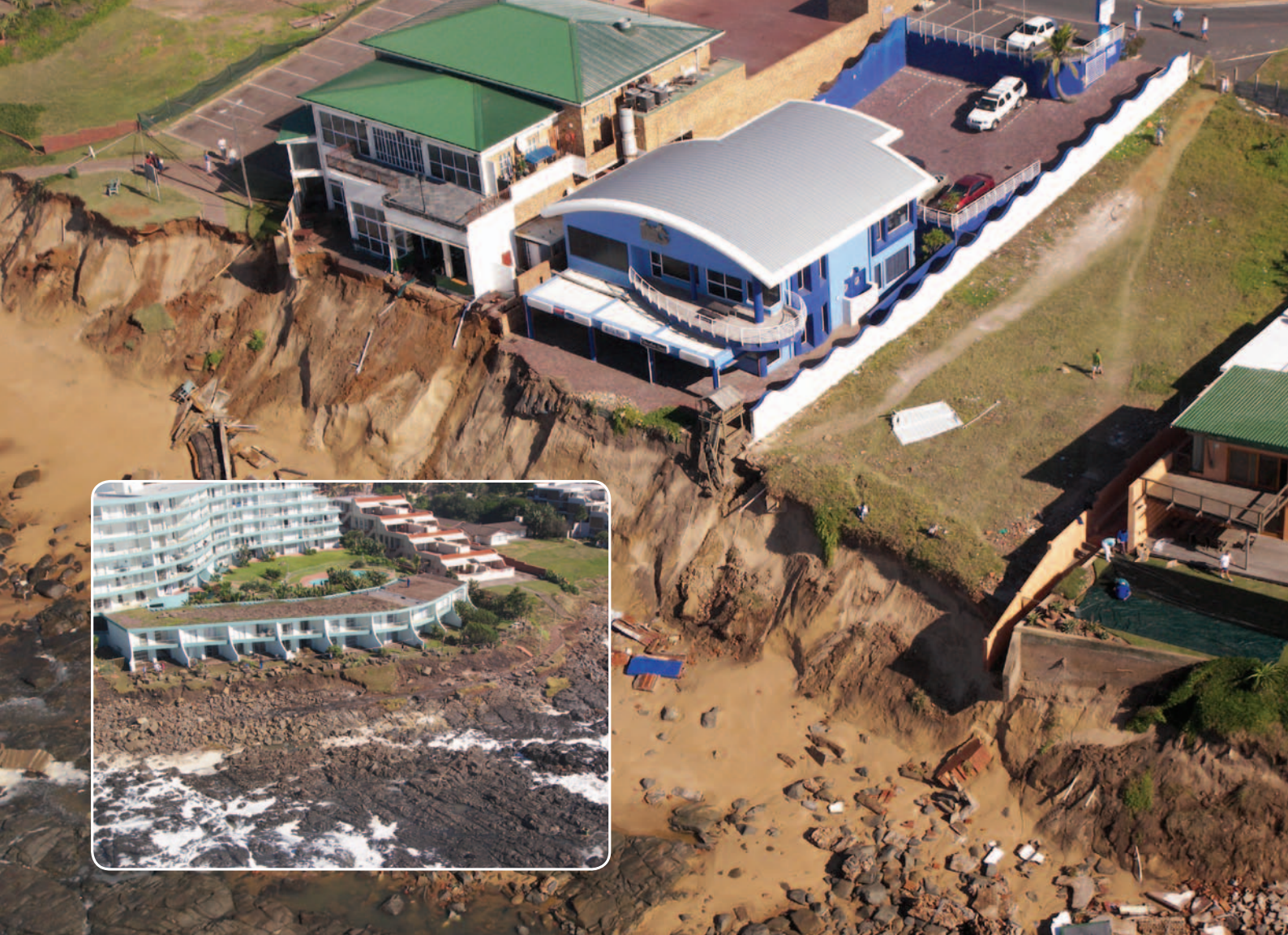
Top left: Coastal erosion at Willards Beach, Ballito after the March 2007 sea storm. Above: Coastal erosion in Ballito after the March 2007 sea storm. Inset: Erosion and property damage in Ballito after the March 2007 sea storm. Photographs: Simon Bundy.
