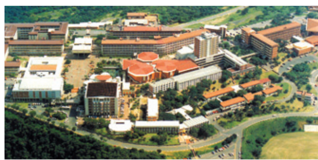
Aerial view of Westville Campus.
